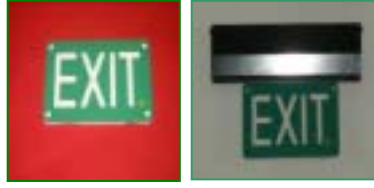
Replaced conventional emergency exit signs to self-luminous type
