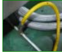
Arrested all compressed air pipe coupling leakages
